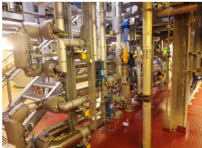
A section of Croda’s new plant at Rawcliffe Bridge
